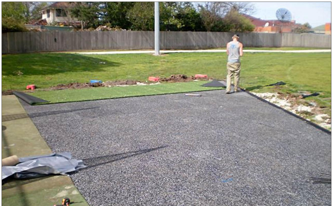
The 20mm shockpad layer completely installed on top of Flo-Cell ® layer.
