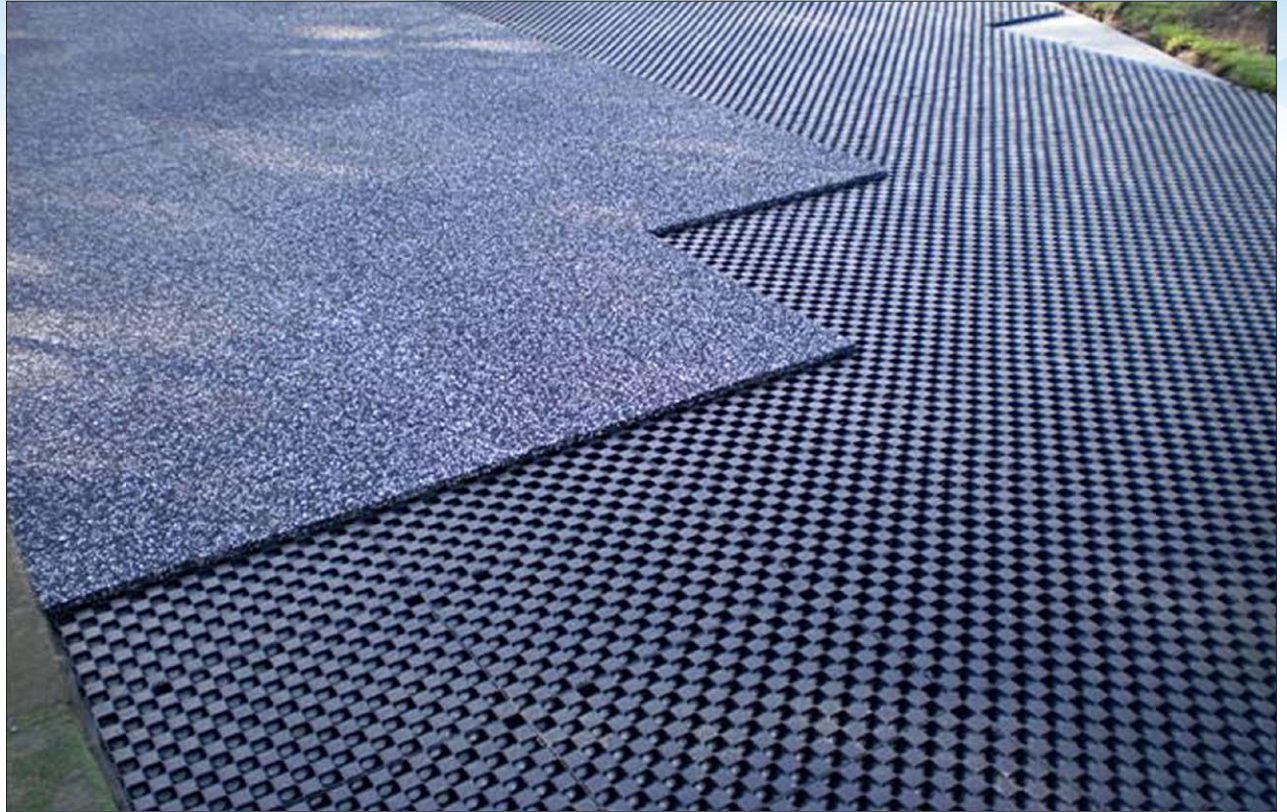
Installing the 20mm shockpads on top of the Atlantis ® Flo-Cell ® layer.
