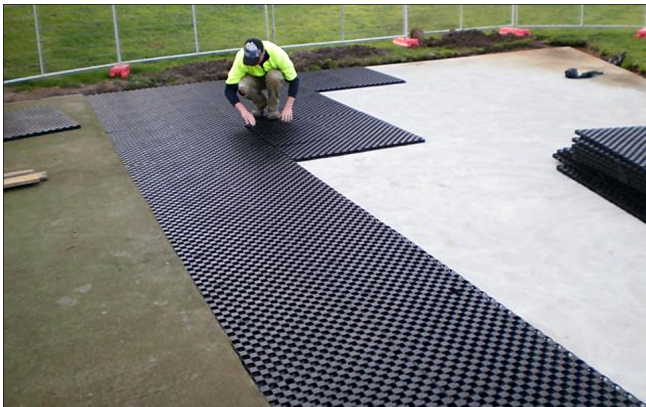
Installing the Atlantis ® Flo-Cell ® drainage cells.
